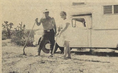
VIC AND JOAN FITZGERALD, SELIGMAN, ARIZ. ARE CLEARING THE GROUND ON LOTS 306 AND 307, MEADVIEW TERRACE, WHERE THEY PLAN TO BUILD AN A FRAME HOME.
