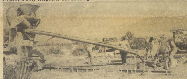
Pouring foundation & floor for Citizens Utility telephone Co new building
