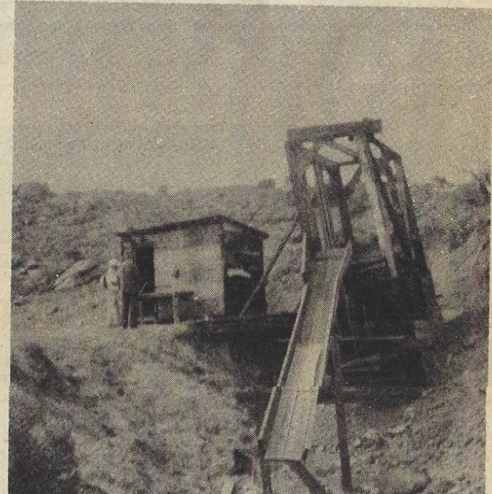
Shack, chute, tunnel and shaft-all together.
