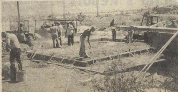
Freiday Construction Co. works on foundation form for new Citizens Utility telephone Co. building.
