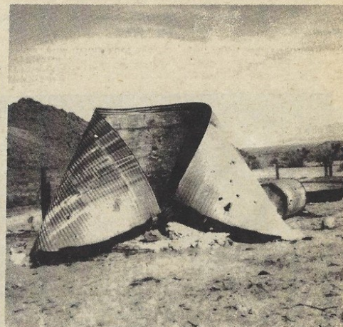
Remnants of large tank, concrete lined inside.
