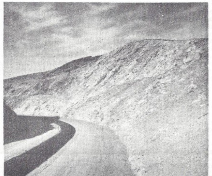
A WINDROW OF ASPHALT WINDS THROUGH THE BIG CUT ON THE SOUTH COVE ROAD.
