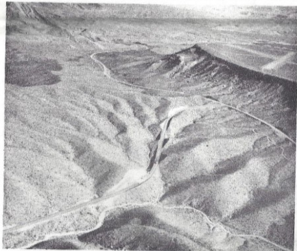
ANOTHER BEFORE AND AFTER PHOTO. ON THE LEFT CAN BE SEEN THE EARLY GRADE AND ALIGNMENT OF THE SOUTH COVE ROAD, WITH PIERCE FERRY ROAD AND THE PIERCE FERRY AIR STRIP IN THE BACK.
