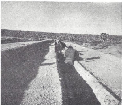
AND THE INSTALLATION.
