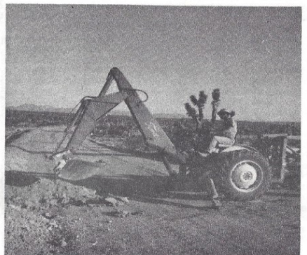
THEN THE SERVICE CONNECTION CROSSINGS.
