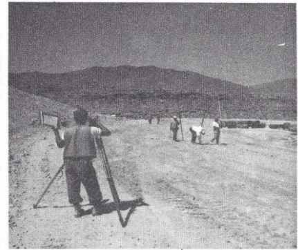
SURVEYORS STAKING OUT FINISHED GRADE.
