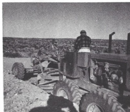
THEN THE FINISHED GRADING COULD TAKE PLACE.
