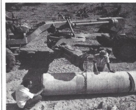
FINALLY, CULVERTS WERE INSTALLED WHERE THE NEW ROADS CROSSED THE NATURAL DRAINAGE WAYS.
