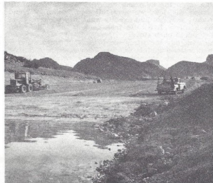
A YEAR LATER WITH THE COMPLETED RAMP. FINISHED GRADING OF THE BANK, OF COURSE, IS YET REMAINING TO BE DONE.
