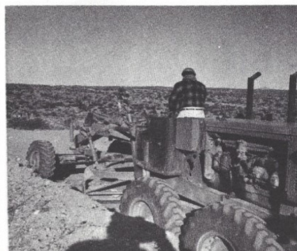
THEN THE FINISHED GRADING COULD TAKE PLACE.
