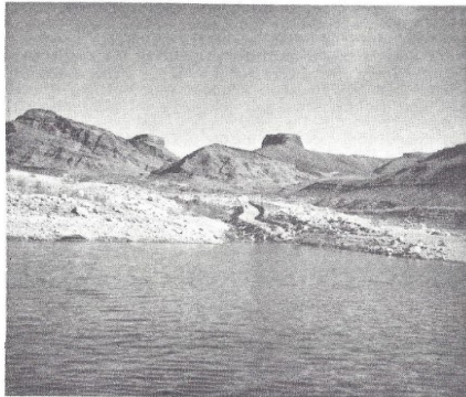
EARLY IN THE CONSTRUCTION PERIOD YOU CAN SEE THE PIONEERED ROAD AS IT MET THE LAKE. IN THE PHOTO AT THE RIGHT, THE SAME LOCATION NEARLY
