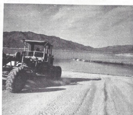
PUTTING THE FINAL TOUCHES TO THE FINISHED GRADE AT THE SOUTH COVE LAUNCHING RAMP.
