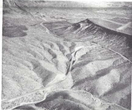
ANOTHER BEFORE AND AFTER PHOTO. ON THE LEFT CAN BE SEEN THE EARLY GRADE AND ALIGNMENT OF THE SOUTH COVE ROAD, WITH PIERCE FERRY ROAD AND THE PIERCE FERRY AIR STRIP IN THE BACK.
