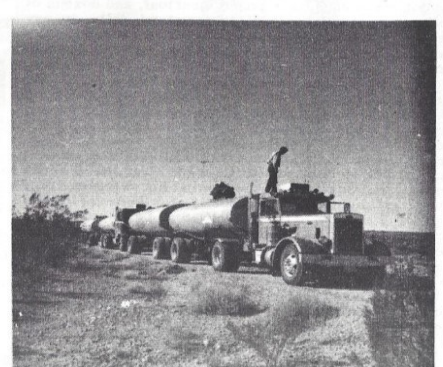
THE FIRST LOAD OF OIL ARRIVES FOR THE PAVING OF PIERCE FERRY RD. AND THE SOUTH COVE ROAD.
