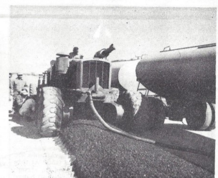
PAVING OF THE SOUTH COVE ROAD IS NEARLY COMPLETED. HERE, EQUIPMENT IS AT WORK, SURFACING A PORTION OF THE PIERCE FERRY ROAD.
