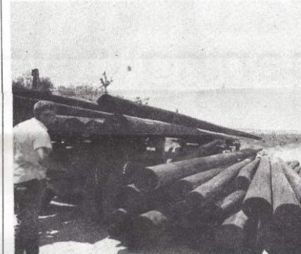
HERE COME THE POWER POLES.
