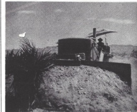
FIRST THE DOZERS HAD TO CLEAR THE ROADBED AND MAKE THE CUTS AND FILLS.
