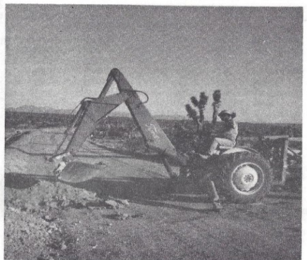
THEN THE SERVICE CONNECTION CROSSINGS.
