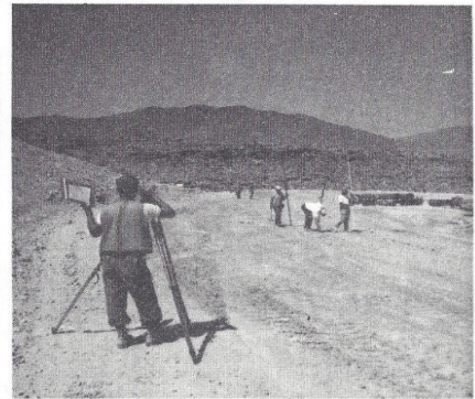
SURVEYORS STAKING OUT FINISHED GRADE.
