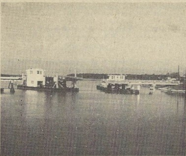
Pontoon bridge on the Intracoastal.
