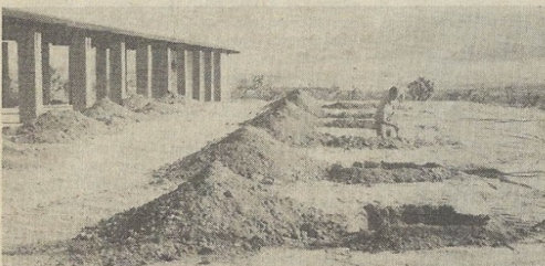
Ditches dug for wing footings.
