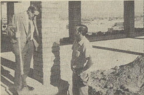
Discussing initial site work.
