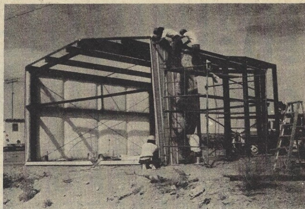
Citizens Utilities Telephone Company building goes up.
