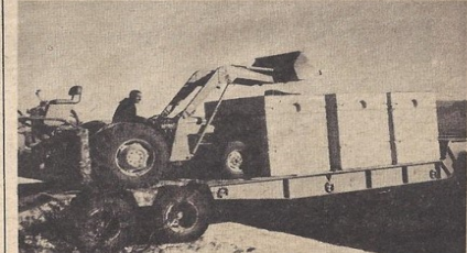
SEPTIC TANKS ARRIVING AT MEADVIEW TERRACE.
