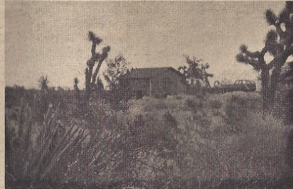
ANOTHER HOME UNDER CONSTRUCTION IN UNIT 3.
